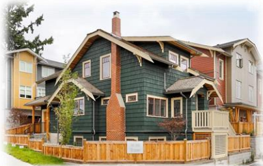
A Haraman project at Roderick Ave, Coquitlam
